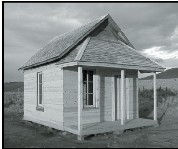
Trout Creek School before and after restoration - 2002.
